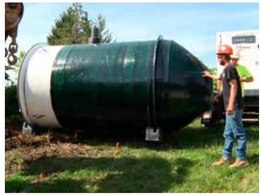
Preparing pump for installation.
