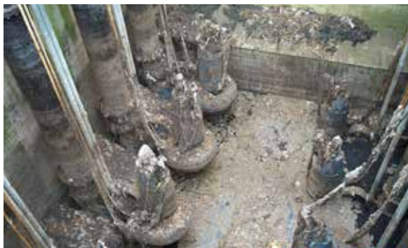
Example of rugs and soft solids developing a surface mat.
