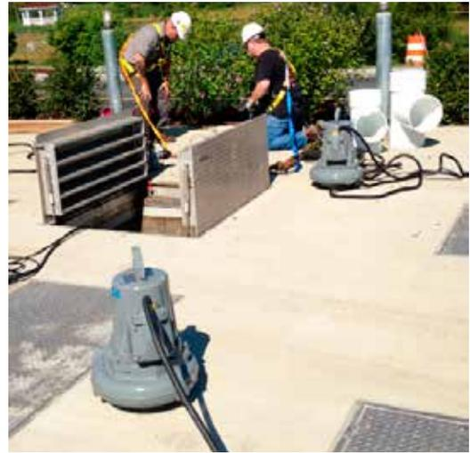
The installation of Flygt brand N-technology impeller pumps.
