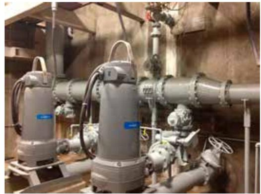
Standard air cushioned check valves and Flygt Pumpsmart VFD's allowed for the elimination of the old style hydraulic oil operated valves decreasing complexity of the system.
