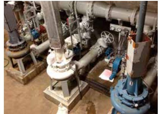
Shafting, coupling guards, seal system, compressor, bearings and hydraulically operated valves required constant maintenance and repair.
