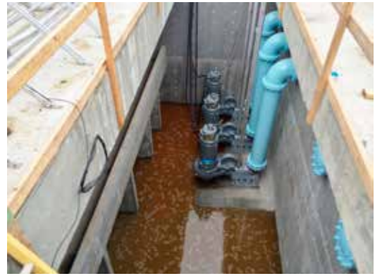
Pumps at the heat exchange facility move water through the NIC loop to the buildings to for use in their heating and cooling systems.
