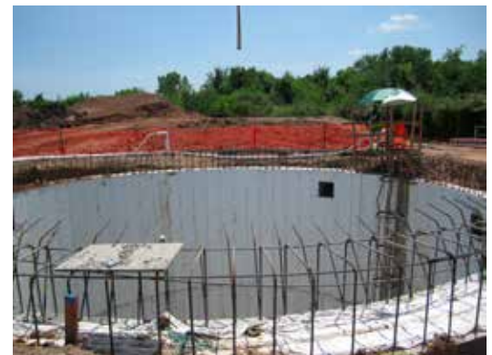
Construction of “Station in the Round” in Sims Bayou
