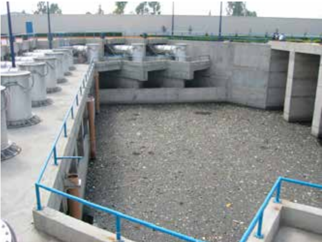
Figure 1: A wastewater sump covered with floating debris.
