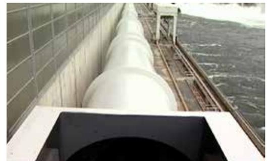
The flow directs the fish into safety through the 9 feet diameter x 4,600 feet long bypass pipe
