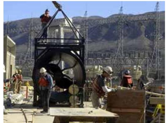
Flygt PK7900 pumps are prepared to be installed in stacks of 3 per each rack
