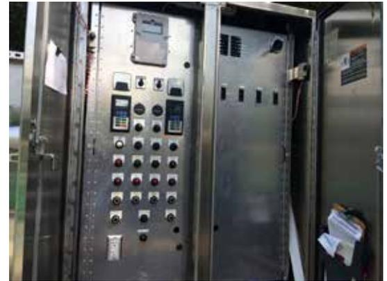
The station was equipped with a 35HP VFD Control.
