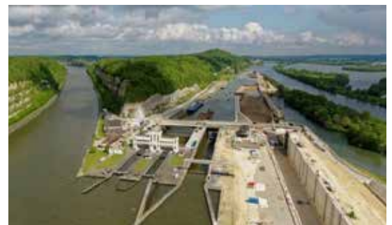
Lanaye Lock #4 being constructed
