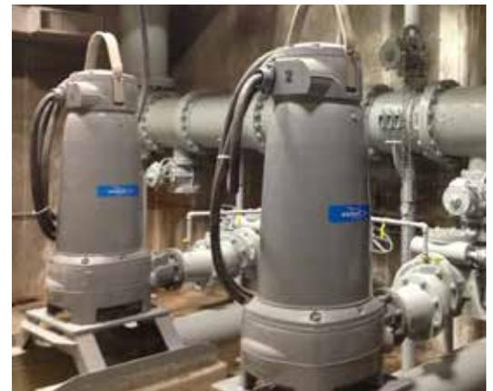
AFTER: Standard air cushioned check valves and Pumpsmart VFD's allowed for the elimination of the old style hydraulic oil operated valves decreasing complexity of the system
