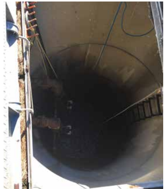
Down in the sump
