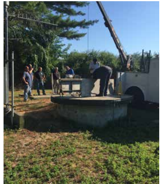
Concertor being installed in the Stony Brook pump station
