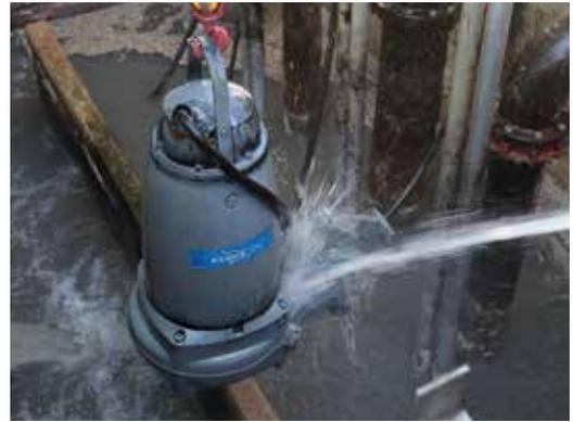
Lifting a Flygt N-pump for a quick rinse.
