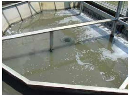
Before: The plant's five floating mixers/aerators could not deliver enough oxygen or mixing.
