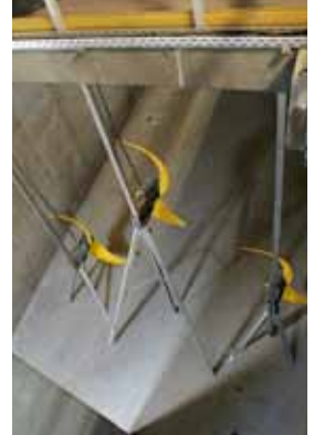
The guide bar system makes mixers easily accessible.
