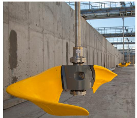
The banana blades help keep the bottom free from sediment and the surface free from floating sludge.
