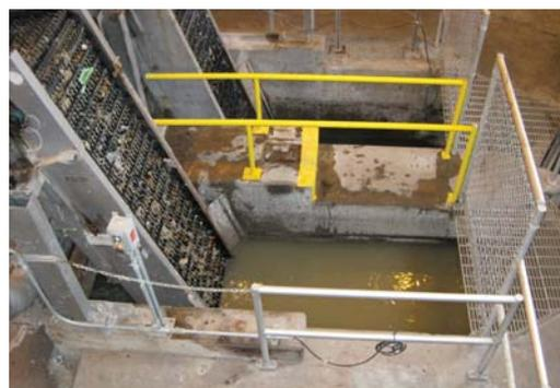
Influent bar screens complement the new influent station pumps, which improve solids handling and energy efficiency.
