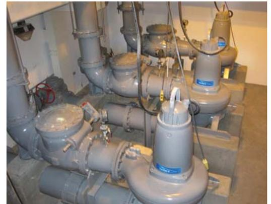
South Adams County Water and Sanitation District (SACWSD) has experienced significant energy savings after replacing aging 60-HP long-shaft pumps with these Flygt 60-HP submersible pumps in a dry pit configuration.
