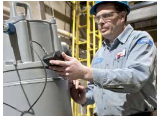
Preparing the N-pump for installation.
