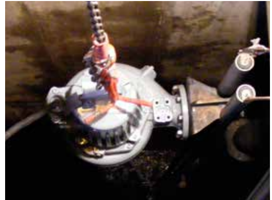
Installing the new N-pump.
